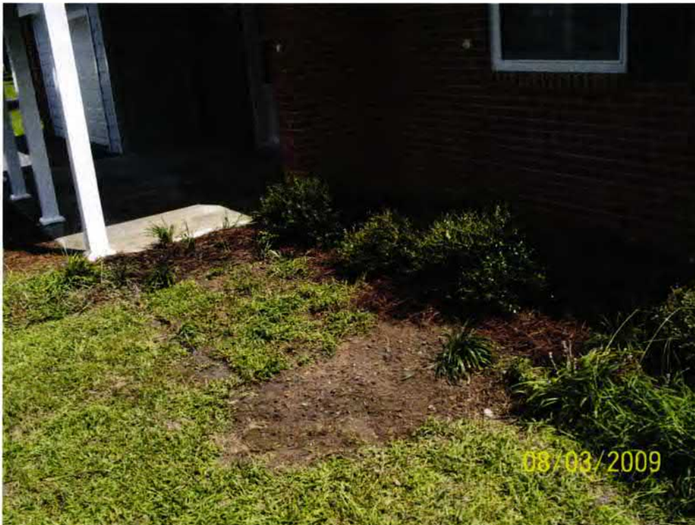
Picture 2: Site after completion of work.
